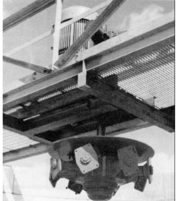
Figure 3 Electrically Operated Variable Pitch Fan
